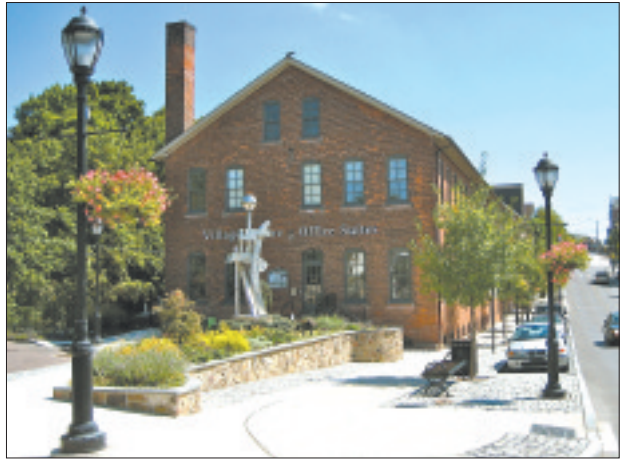
The Souderton office suites are on the National Register of Historic Places.
